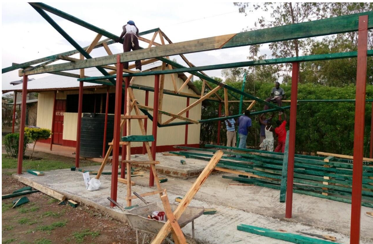
Bouw Multi Purpose Hall
